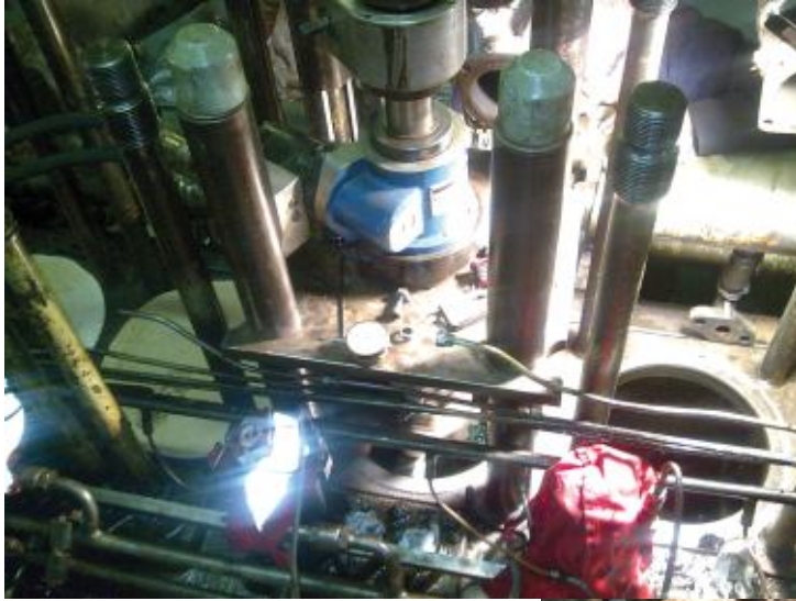
Machine Set Up & Work In Progress
