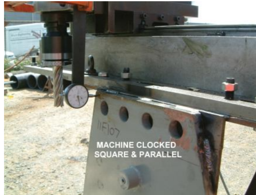
On-site Machining of incorrectly manufactured support leg.
