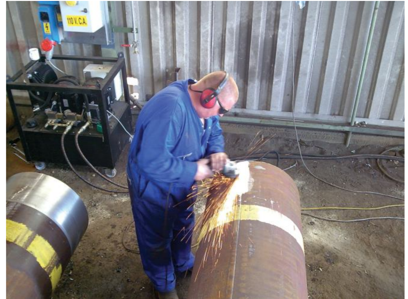
Grinding In Progress
